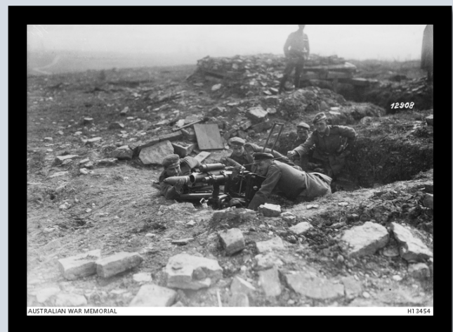
Figure 2. A 7.6-cm minewerfer , or 'mine-thrower', on a new model carriage incorporating a trail and spade that allowed flat trajectory fire for the engagement of tanks. This photograph, donated to the Australian War Memorial by the German War Museum, is captioned October 1918. The casual attitude of the onlookers, and the lack of steel helmets and camouflage, suggests that the photograph was taken well behind the front-line, possibly at a school. (AWM Collection H13454)
