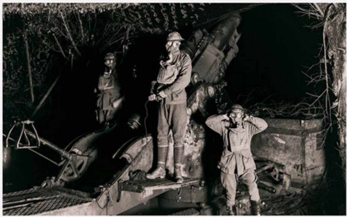
Above: Gunners of the 36th Siege Artillery Group, with a 9.2 inch howitzer, the heaviest gun operated by the RAA, with a range of 9,000 meters for it's 130kg shell.
